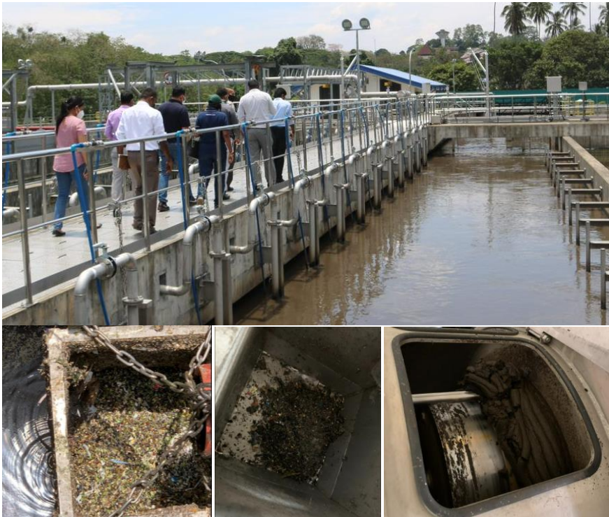
WASTEWATER TREATMENT PLANT: KANDY
